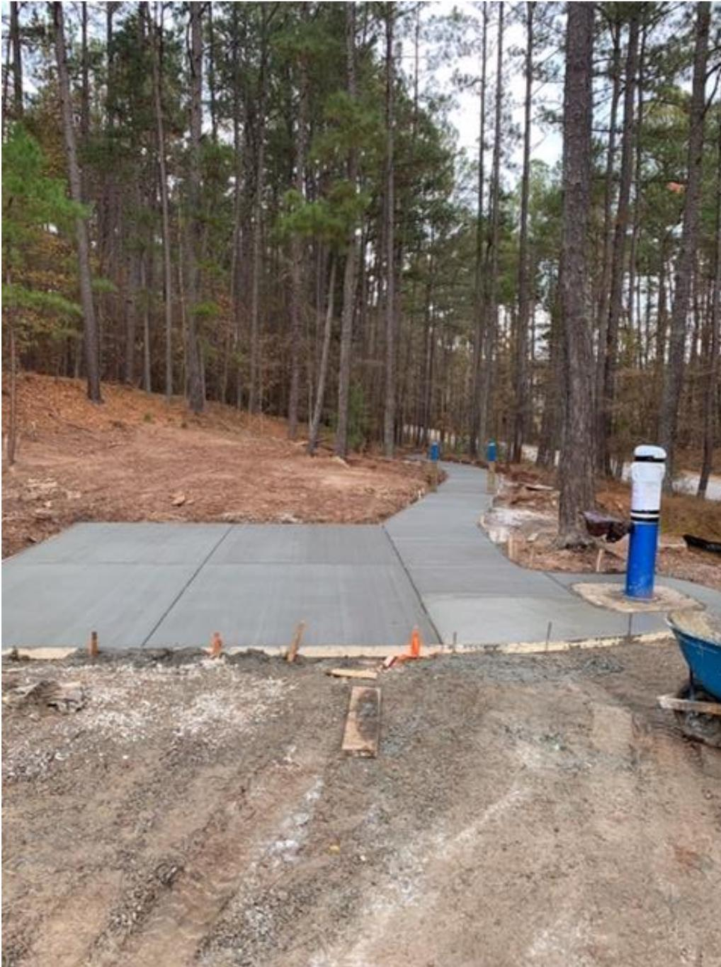
View of Parking Space, Aisle and Connector at Pittard Sears Shortly After Concrete was Poured in early December 2018
